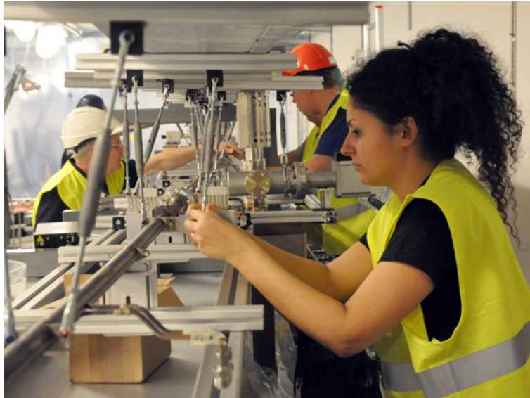
The 3 GeV ring vacuum system under installation in 2015.
