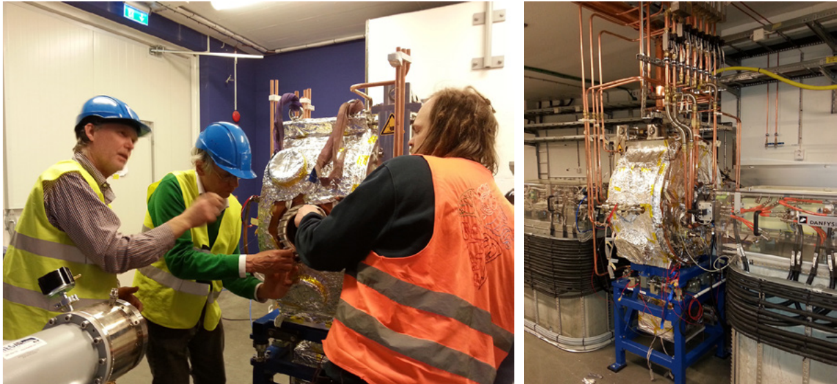
Installing the power coupler in a 3 GeV 100 MHz RF cavity (left) and the final installed setup (right) in the 3 GeV ring.
