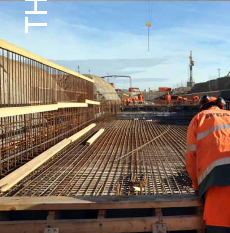
2. Assembly of the steel reinforcement bars for the slab and walls in September 2011.
